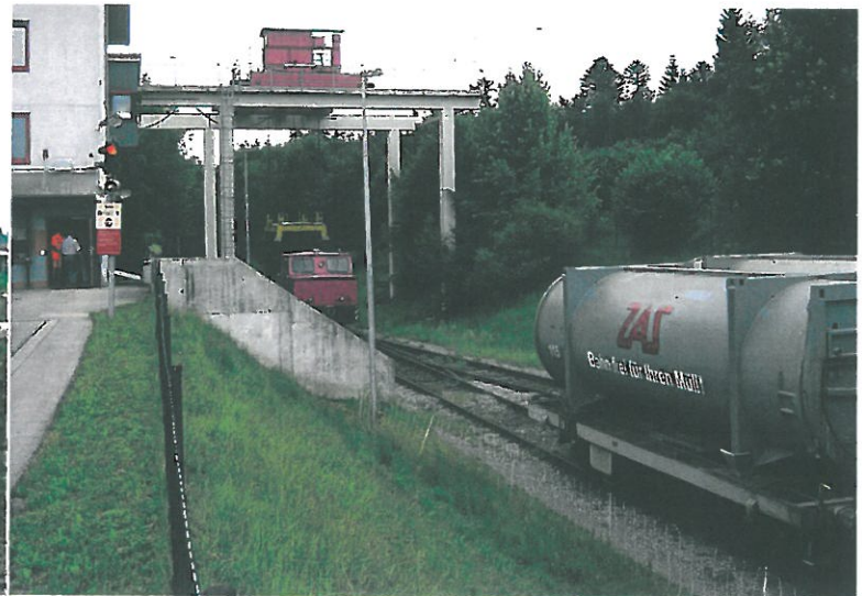
Müllumladestation ZAS Weiderting
